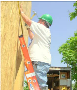
Greg Young nails on siding.
